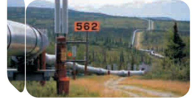
Pipeline for NICO
